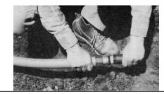
**6.** Tighten assembly by holding body with one wrench and turning nut with another.
