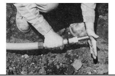
**5.** Insert pipe with components into body. Slide riser casing forward and thread nut onto body.
